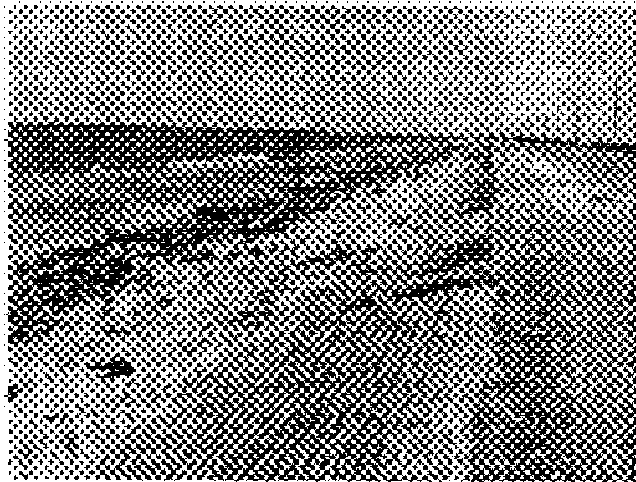
Figure 15. Gobi block revetment, Holly Beach, LA
